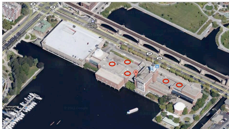
Fig. 5. Red circles show location of anemometers on rooftop of Museum of Science, Boston.
